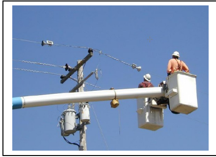
INSTALLATION OF E-LINE ANTENNA NODE
